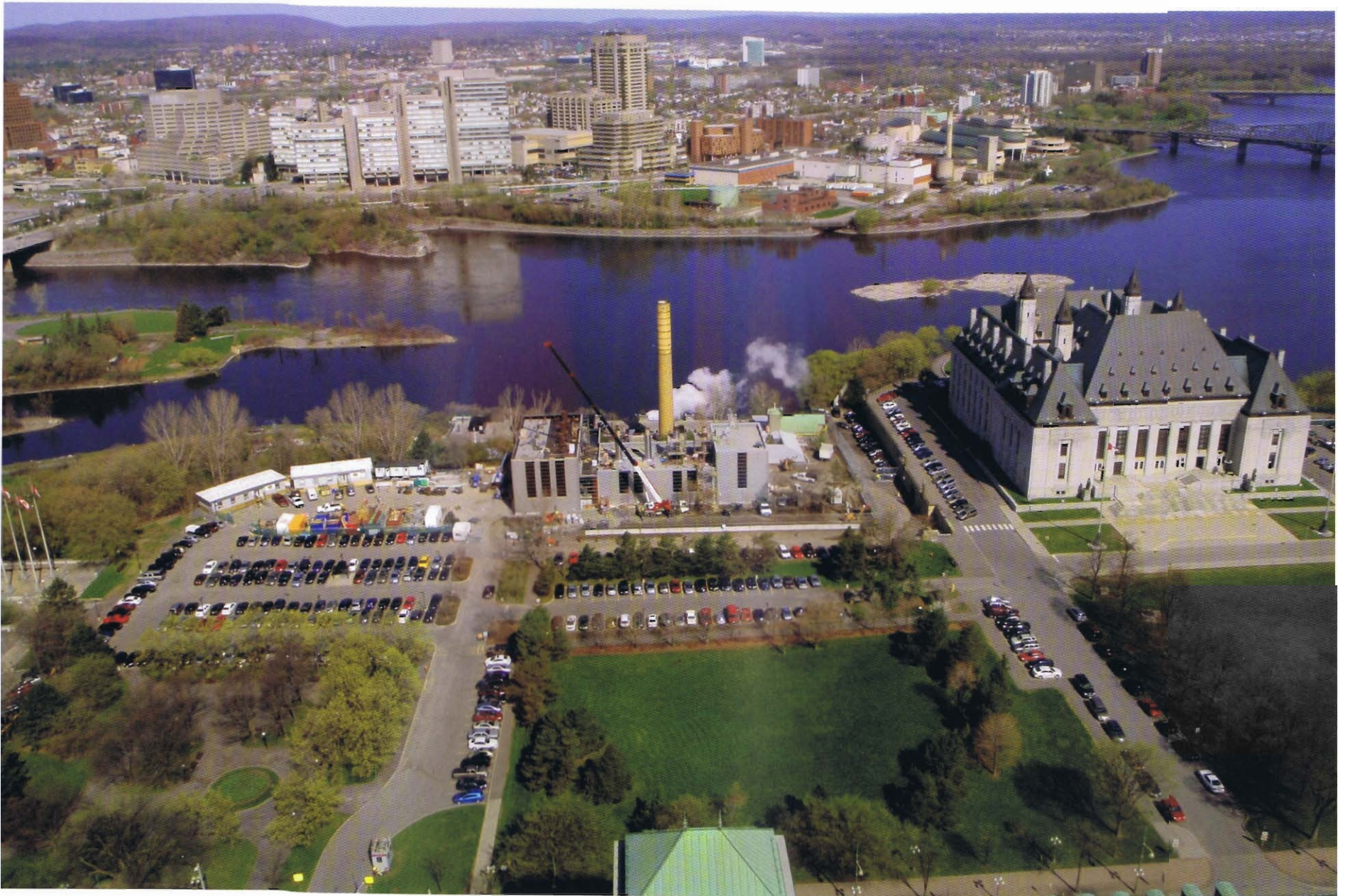
Day 79: The steam blow process from afar.
